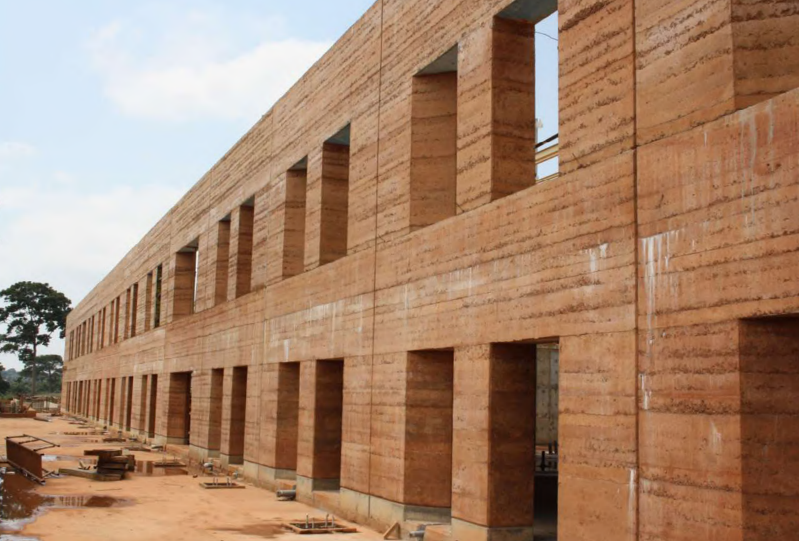
01. Vista prospetto ovest | West elevation view Photo by Emergency Archive
