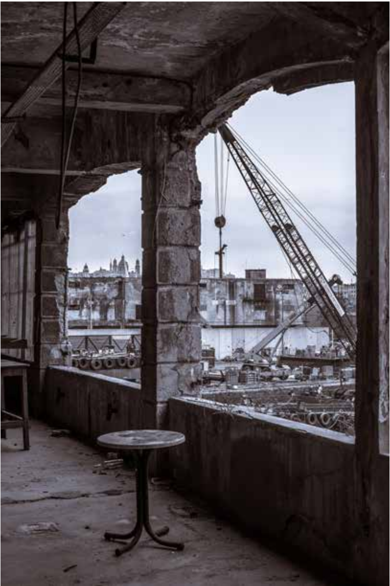
Ex silo granaio Hennebique, viste interne Former grain silo Hennebique, internal views Gianluca Porcile, 2015
