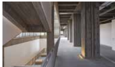
La galleria esterna degli spazi espositivi con la struttura in cemento a vista The external gallery of the exhibition areas and the Reinforced concrete structure on sight Photo © Ali Bekman
