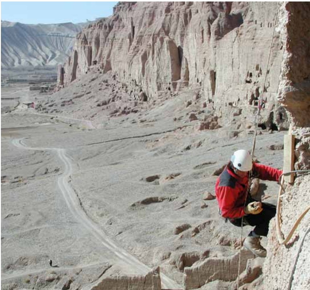
Lavori in corso durante la campagna di consolidamento, 2003. Foto C. Margottini (in alto) Works in progress during the consolidation campaign, 2003. Photo by C. Margottini (above)
