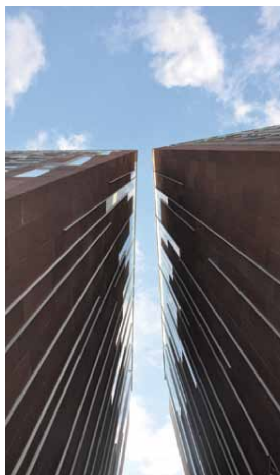
Überseequartier, residenze e uffici Sumatra, cantiere (in basso a sinistra) e distanza fra i blocchi (a destra), EEA Erik van Egeraat associated architects, Rotterdam. Foto Barbara Frediani-Gasser Überseequartier, homes and Sumatra offices, site (below on the left) and distance between blocks (on the right), EEA Erik van Egeraat associated architects, Rotterdam. Photo Barbara Frediani-Gasser
