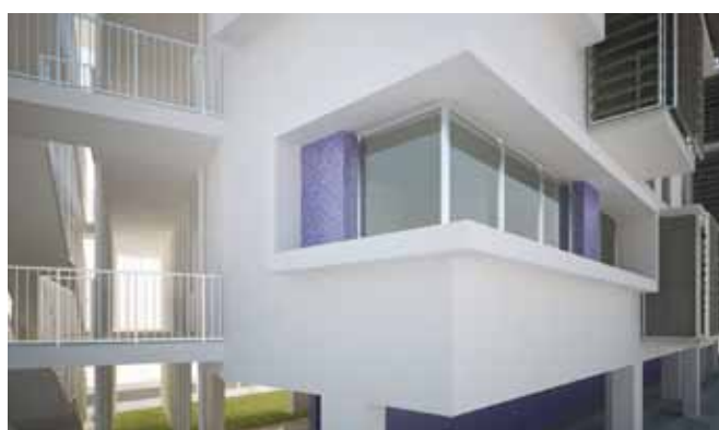
Dettaglio del fronte Sud e vista del giardino condominiale Detail of the South front and view of the common garden
